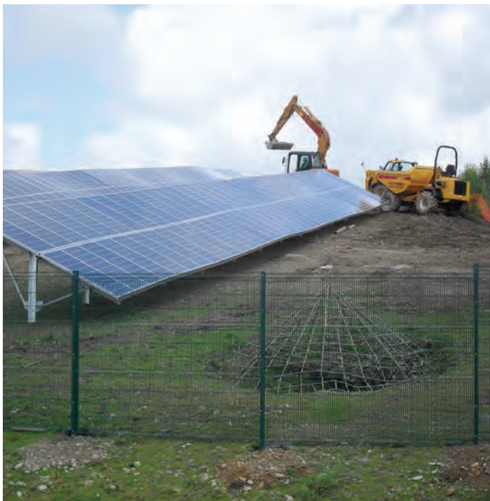
Figure 5 Construction of a 1.4MW solar farm at the former tin mine site at Wheal Jane, Cornwall. Such sites should generally be considered for such development in preference to agricultural land.
