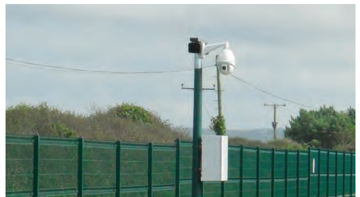
Figure 12 Any security equipment, such as this CCTV system, should be as discrete as possible in order to minimise its visual and landscape impact.
