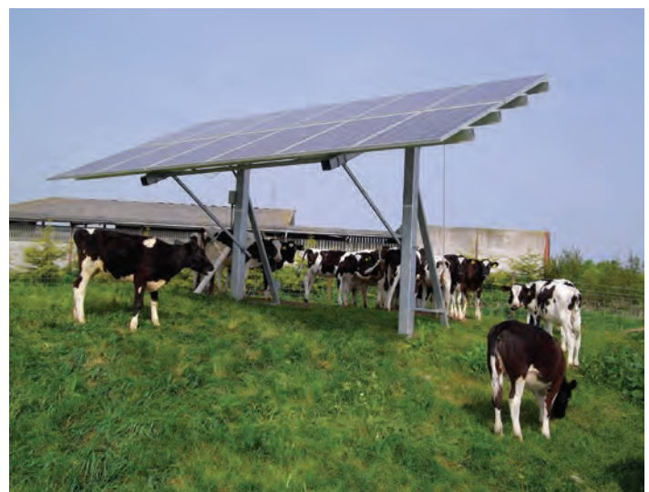
Figure 4 Sheep and cattle grazing under solar panel arrays. Support structures, and the height of panels, would need to be substantial in order to allow cattle grazing and would not ordinarily be recommended. Images courtesy of Steve Edmunds, Mole Valley Renewables.
