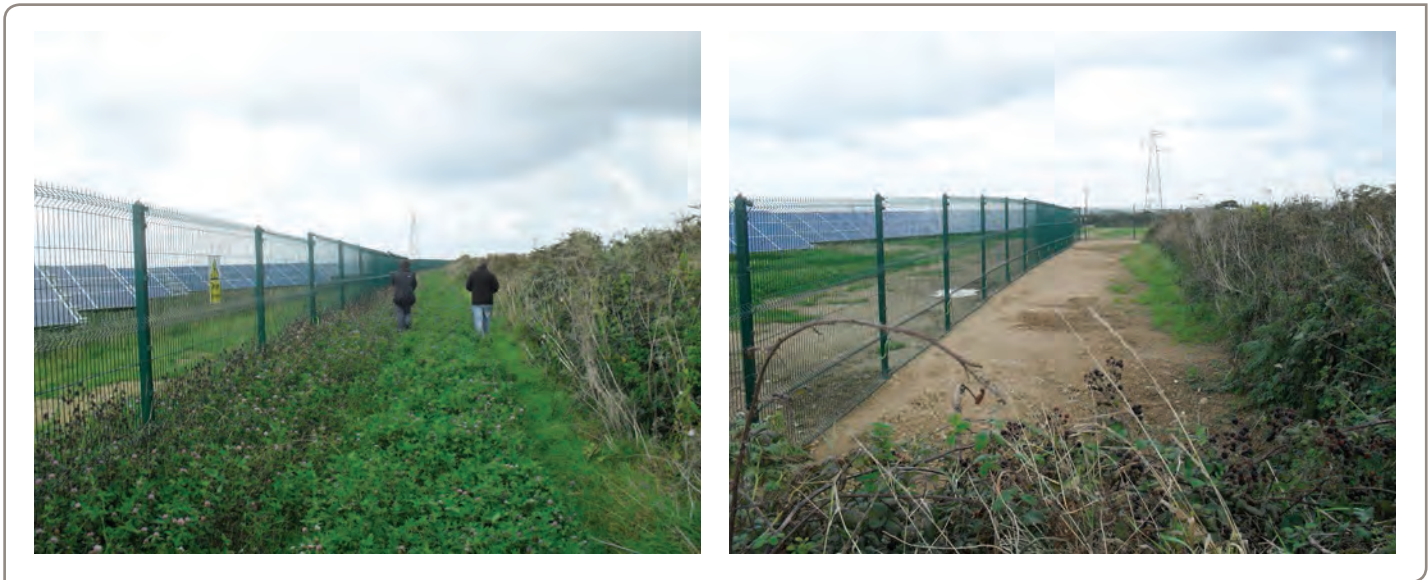
Figure 22 A 5m buffer strip between the field boundary and any fencing will allow access for maintenance purposes, minimise damage to the field boundary and provide an access corridor for wildlife.
