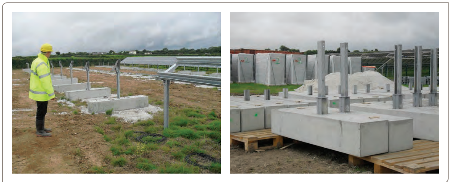
Figure 15 Where there are areas of archaeological interest, and therefore a need to avoid ground disturbance, the use of pre-cast concrete anchors should be considered, as shown here at the 5MW Trefullock solar farm in Cornwall.
